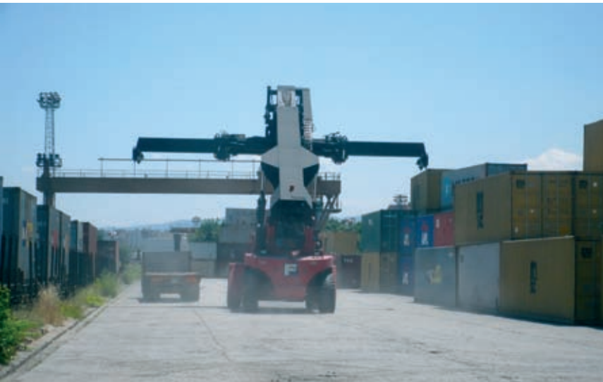
No room for lots of traffic. Cramped conditions, badly maintained infrastructure and a defective portal frame complicate optimum freight handling in Sofia. Photo by Lars Deiterding
